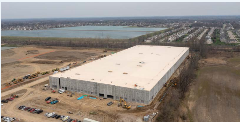
ATS Industrial Automation, Columbus, Ohio
