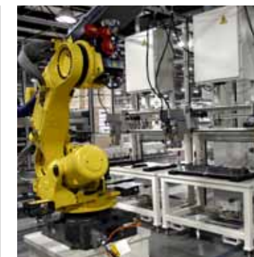
Battery process development for a new product that involves module processing and specialized equipment
